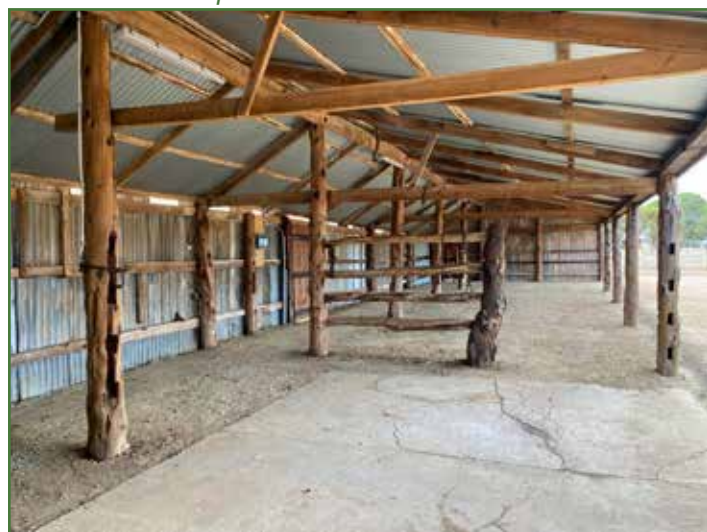
The renovated Stables
